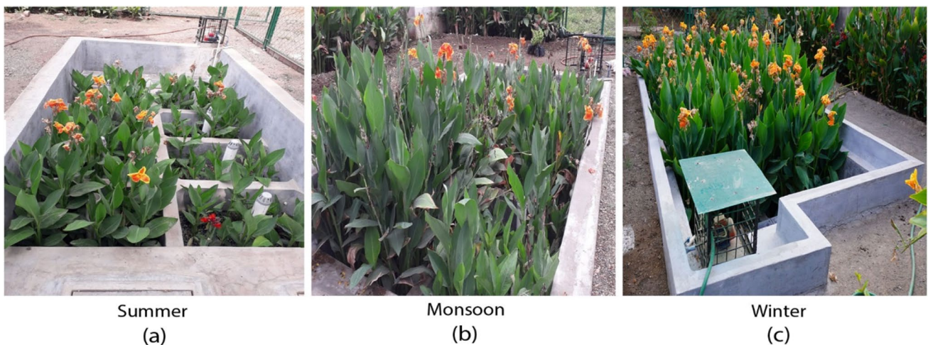
Fig. 2 Wetland system photograph treating residential wastewater a summer (April 2021); b monsoon (June 2021); c winter (November 2021)
